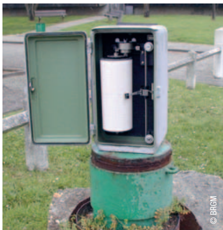
Piezometer used for continuously measuring the variations in groundwater levels.
